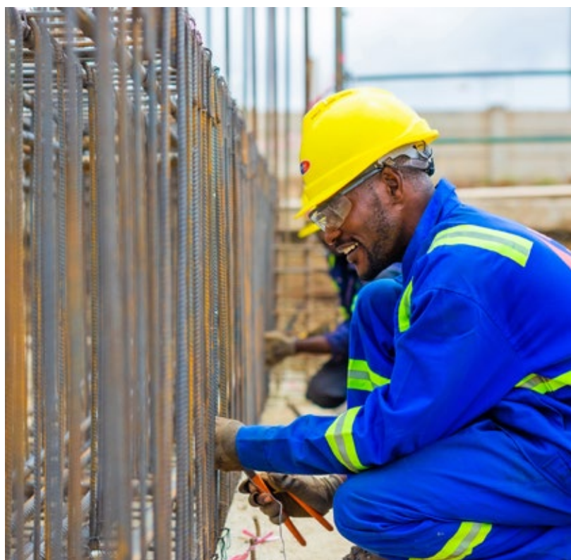
CBI, cement production in Ghana.
